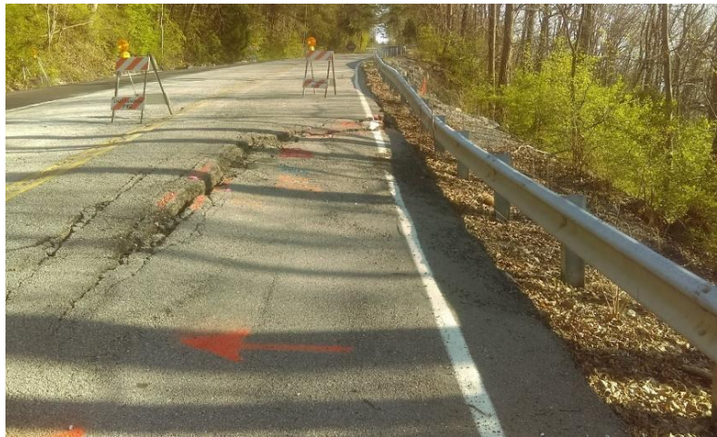
Slope failure
